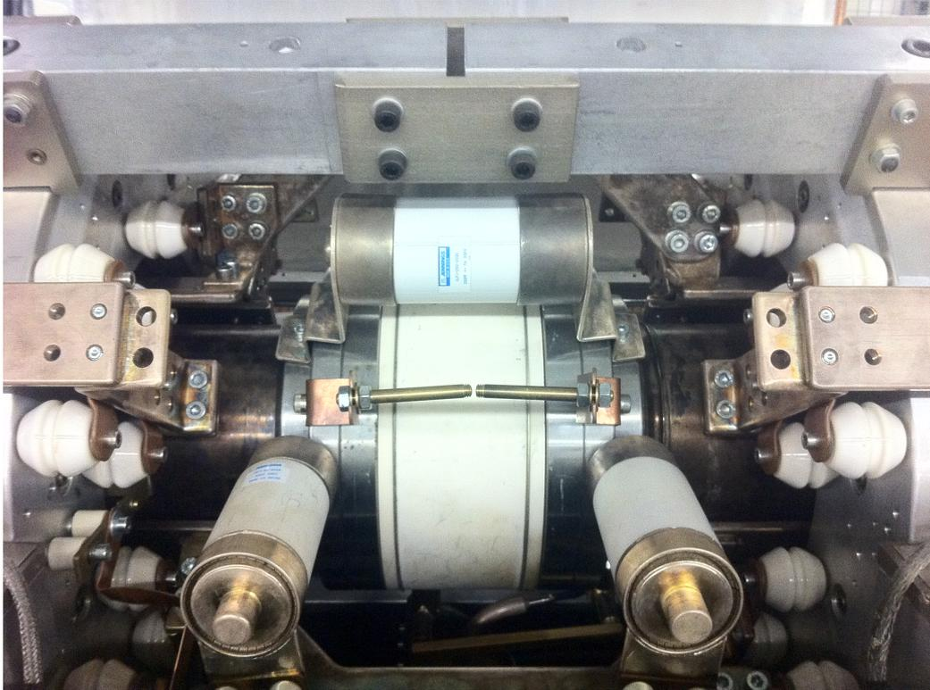
Figure 7.3: *Gap of the SIS 18 Prototype Cavity: In the middle there is the spark gap realized by two lances (gap distance 5 mm). Behind this there is the ceramic gap of the cavity in white dividing the beam pipe.*
